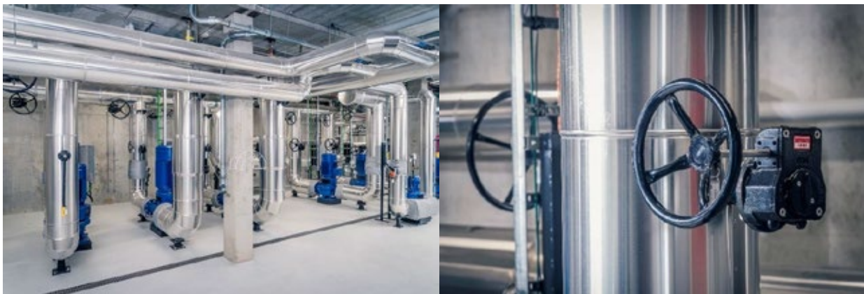
BROEN Ballomax® ball valves controlling the flow of district heating water
