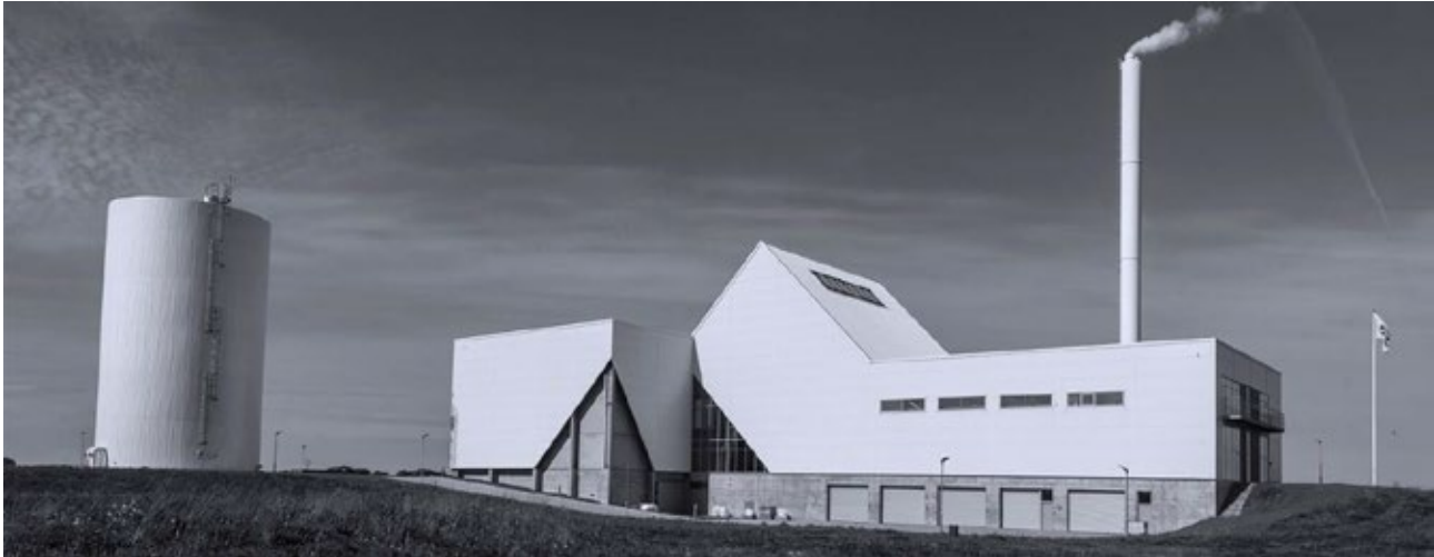
Aabybro district heating plant (Denmark).
