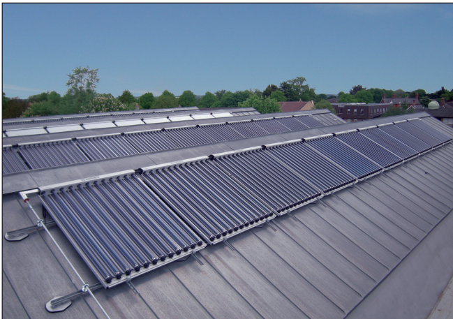
Fig. 49: On-roof mounting with vertical collectors
