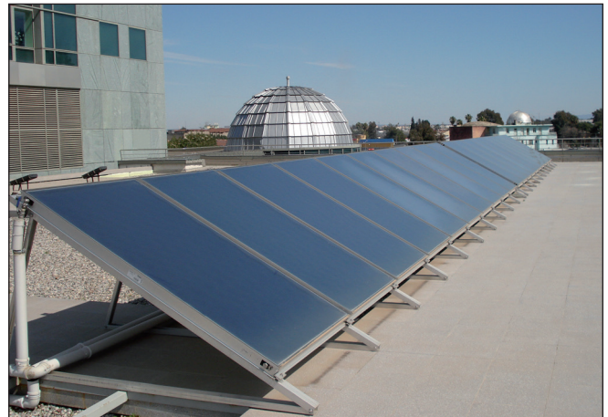
Fig. 50: Vertical flat roof installation
