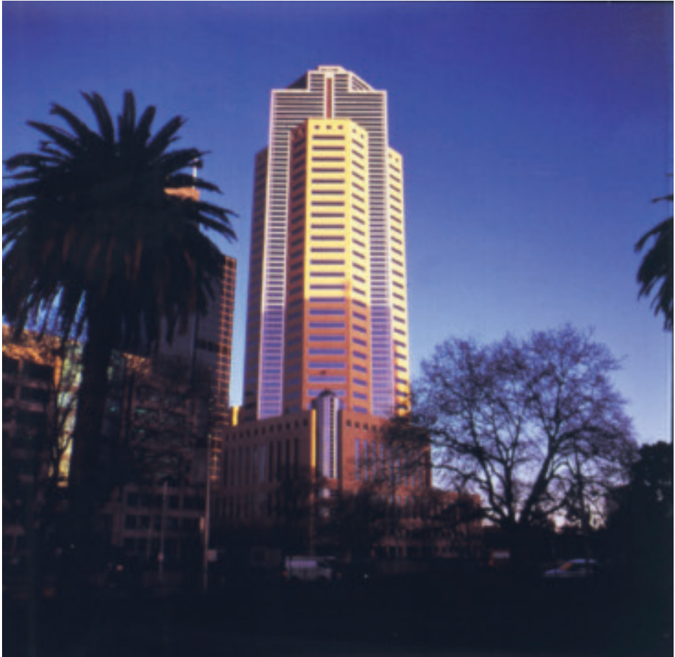
Casselden Place, Melbourne, Australia
