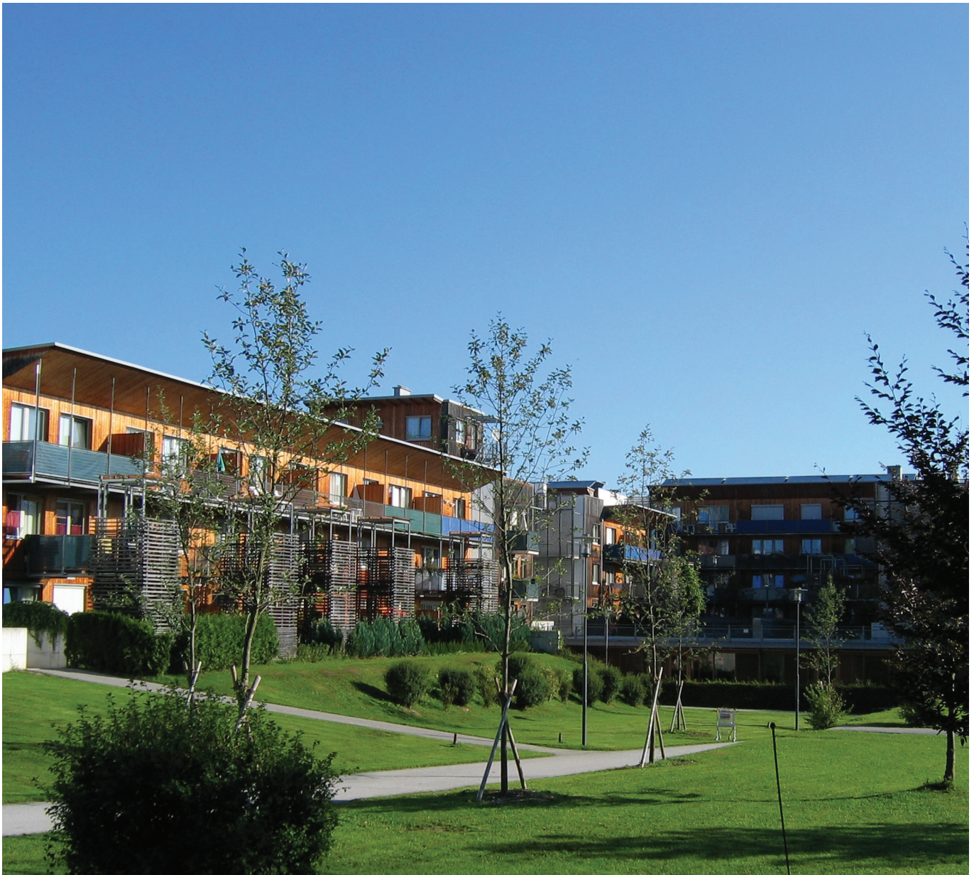
Salzburg, Austria – Multi-family buildings with district heating inside.
