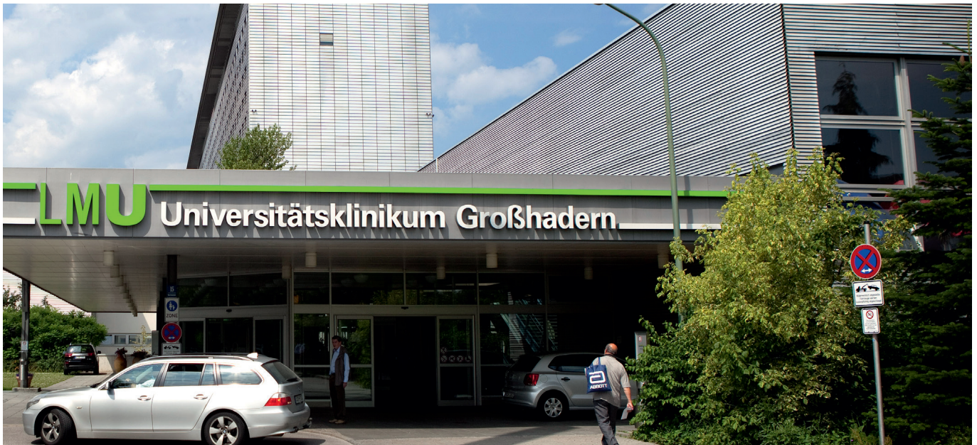
Munich, Germany – Commercial building with heating and domestic hot water production.
