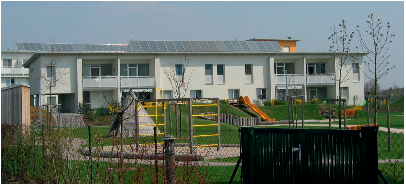
Linz, Austria – Multi-family buildings supplied with district heating.
