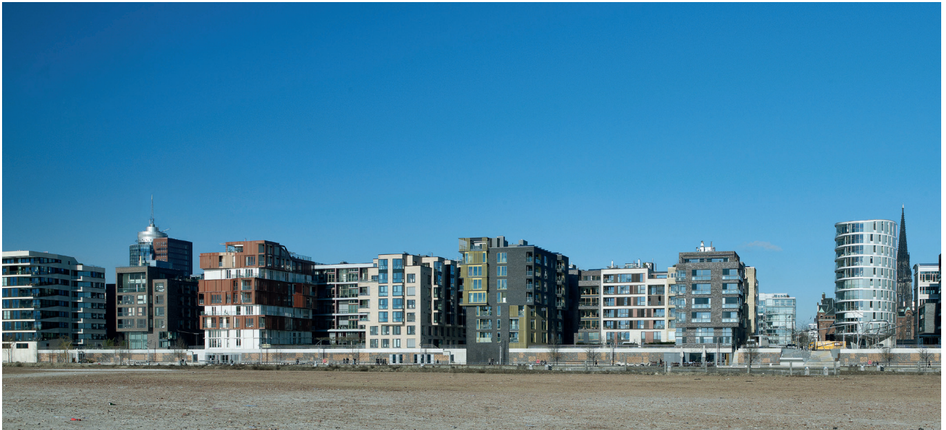
Hamburg, Germany – Multi-family and commercial buildings with heating and instantaneous domestic hot water production.
