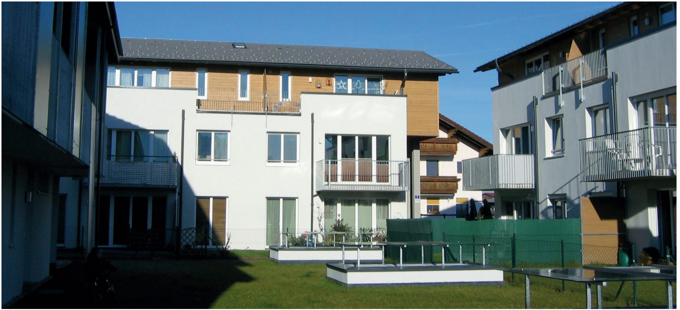
Walz, Austria – Multi-family buildings with district heating inside.
